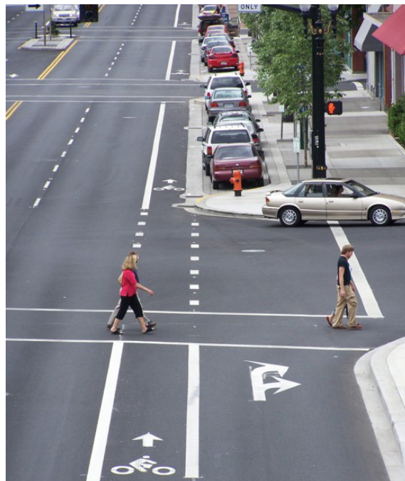
Above two: Complete Streets with on-street parking and Class II Bicycle Lanes
